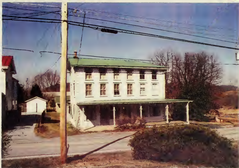
Fig. 124 The old Byers Hotel, now a private residence. Photograph by the author, 1995.
